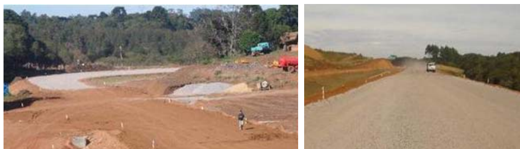
Proving Ground construction works
